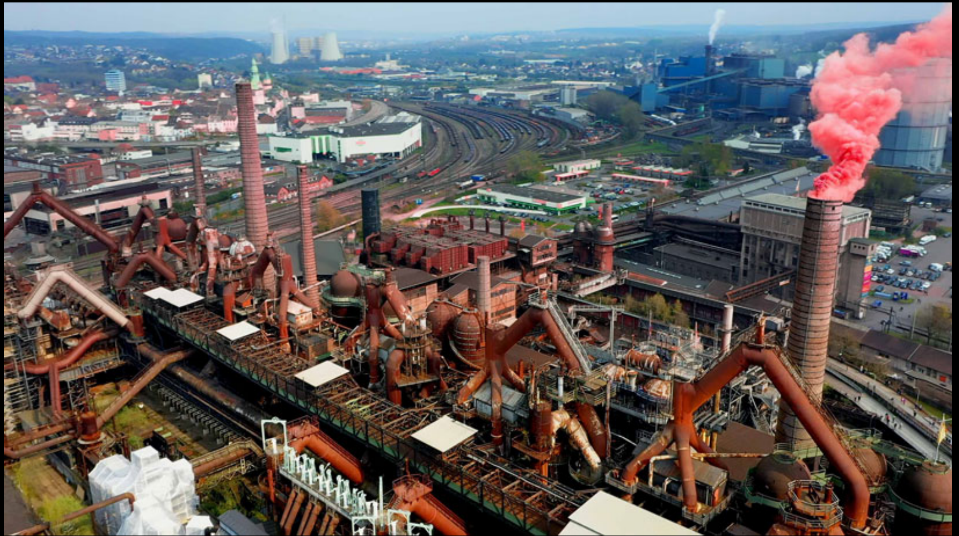
Völklingen Ironworks, Saarland, Germany
